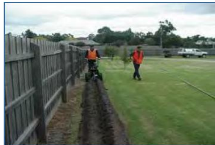
Installing a low pressure grinder pump rising main in private property.
