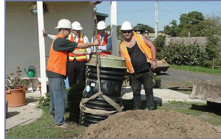
Lowering the unit into position
