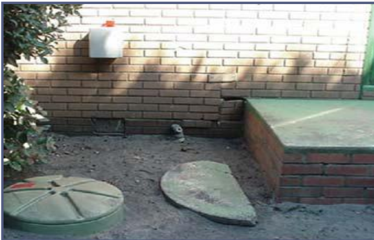
Installation of pump unit & switchboard completed.
