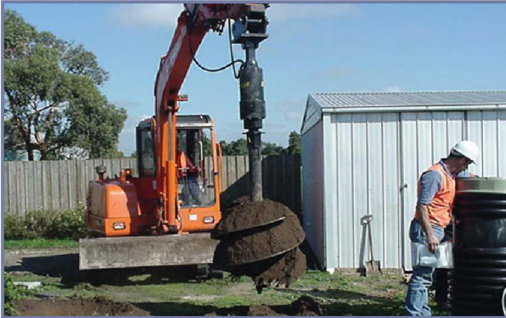
Installation by auger
