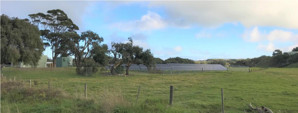
A view of the panels from Toorak Rd, Inverloch
