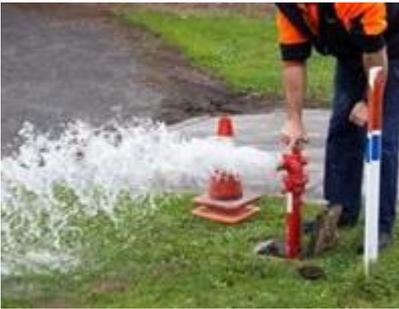
Mains flushing and air scouring is conducted regularly to keep pipes clean.
