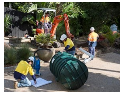
Installation of a Collection Tank
