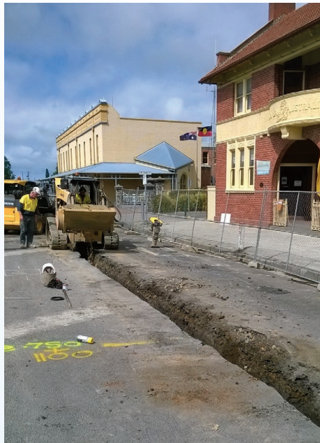
Workers lay the new water main in Commercial Road Yarram
