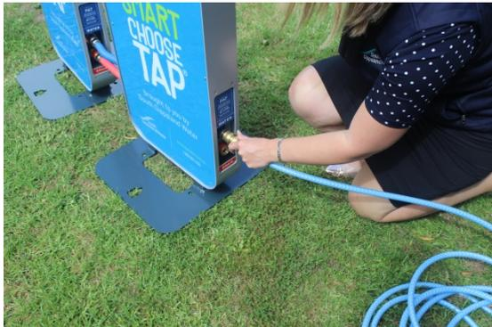
**Step 7:** Connect the red drain hose to the red drain outlet. The drain outlet can be connected to either side of the unit. Position the drain hose towards a drain or garden and ensure it won't be a tripping
