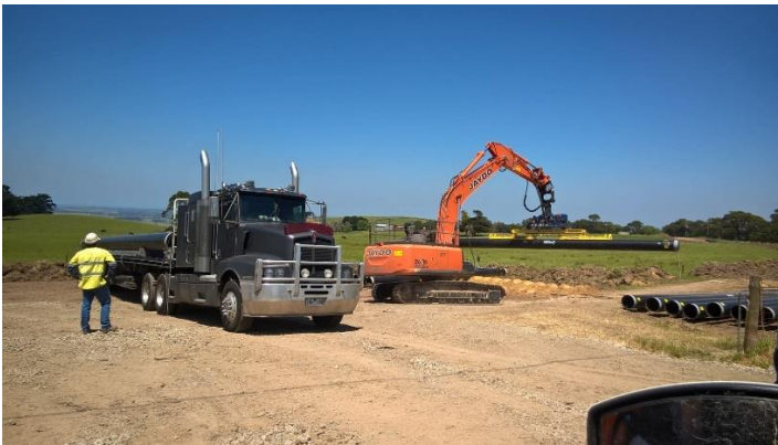
Left – An interesting use for a vacuum. These 1.3 tonne pipes are held by suction for secure unloading and distribution. Right - Locating fibre optic cables along the pipeline alignment
