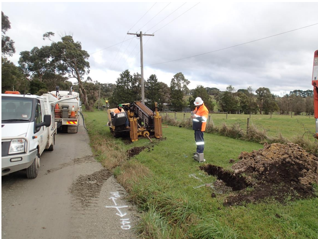
Image: A directional drilling rig in action at Nyora
