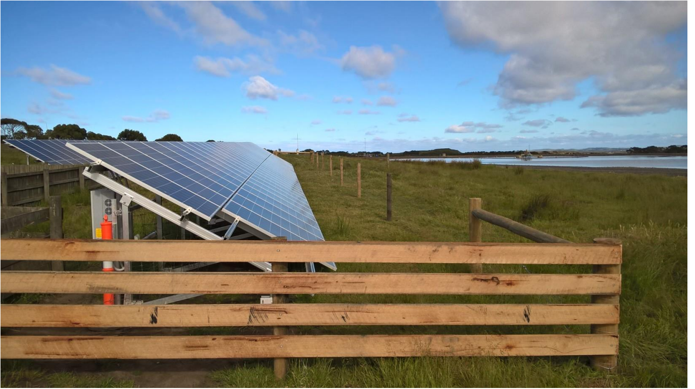
Pictured: Solar Panels installed at Wonthaggi Wastewater Treatment Plant [END]
