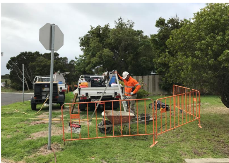
Photo: SGW staff inspecting local infrastructure
