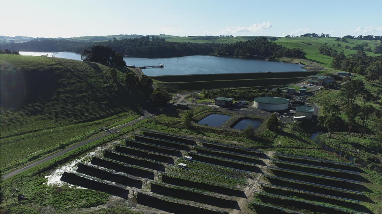
PICTURED: Aerial of Lance Creek Water Treatment Plan
