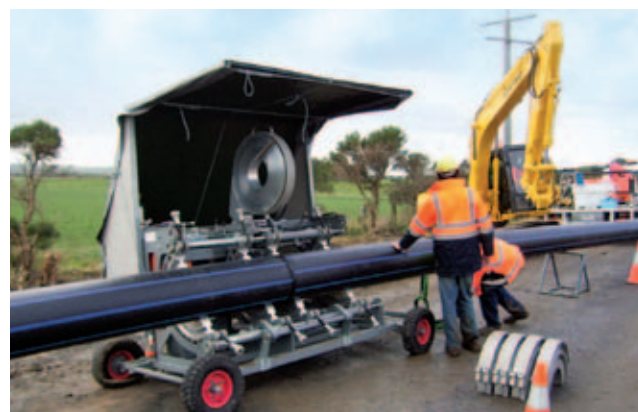
Polyethylene welding equipment in action on the Lance Creek pipe line.
