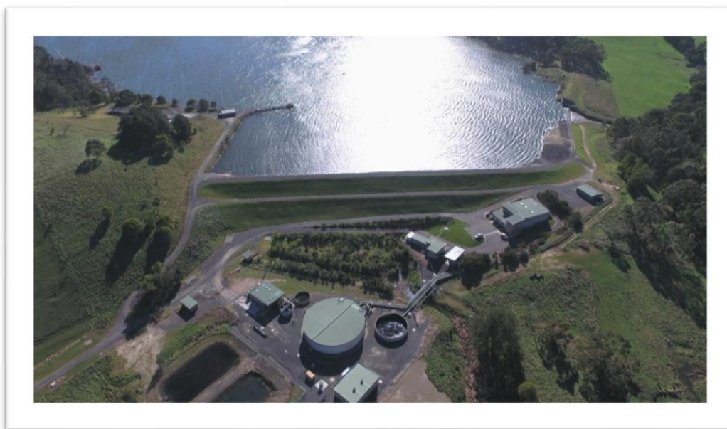
Photo: Aerial view of Lance Creek Water Treatment Plant and Reservoir
