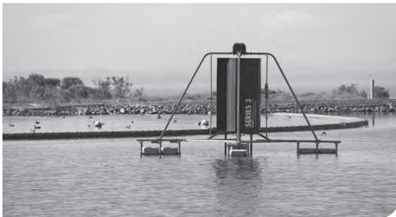
Innovative wind powered mixer installed at the Inverloch Wastewater Treatment Plant
