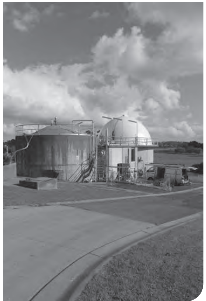
Bio-Dome Leongatha Wastewater Treatment Plant – For gas capture & re-use
