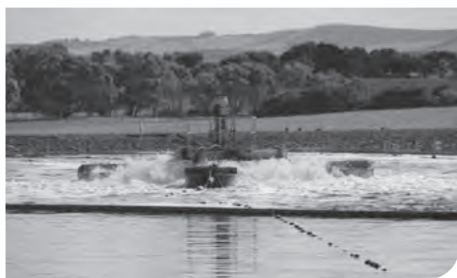
Wastewater lagoon surface aerator
