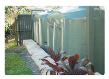
The tank itself needs regular external inspections for leaks and an internal inspection for sludge every few years. This can be dangerous so contact a professional if you need help doing this.
