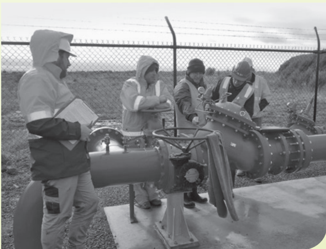
Commissioning of DP5 valve which connects Lance Creek Reservoir to the Desalination Plant and Melbourne Water Supply System. L to R: James Russell (KBR), Dean DeMenech (SGW Project Supervisor), Colin Kirkland (Bermad Valves), Denis Landron (Westsure), Kelvin Staley (Kelcon).
