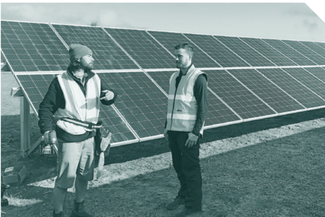
75.6kW Solar system installed at the Lohr Avenue Sewer pump station at Inverloch. It will produce 87% of the sites energy needs.
