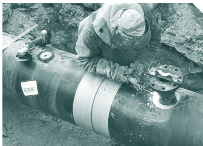
Welding of pipeline as part of the Lance Creek Water Connection.
