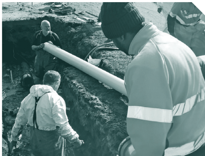
South Gippsland Water's Maintenance Team repair a broken main.
