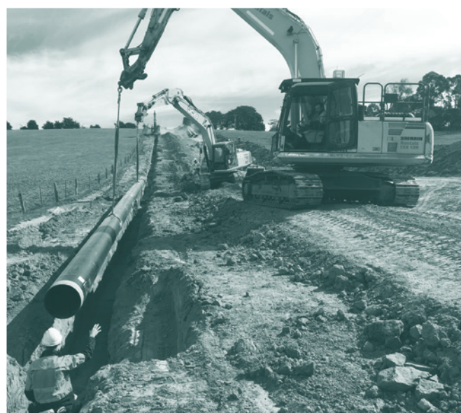
Pipe being laid for the Lance Creek Water Connection and the steep terrain of the pipeline alignment.
