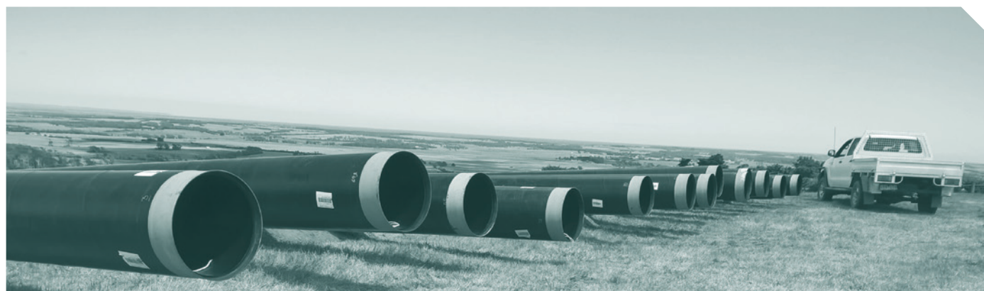
A pipe laydown area as part of the Lance Creek Water Connection project construction.
