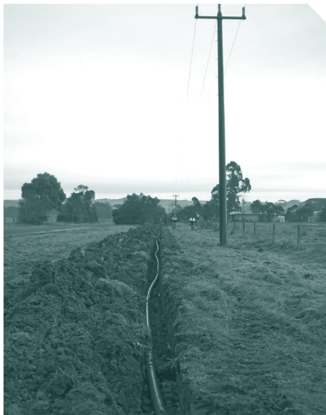
Installation of the new 'purple pipe' that will feed recycled water into Foster from the Wastewater Treatment Plant for re-use at the recreation reserve or golf club.
