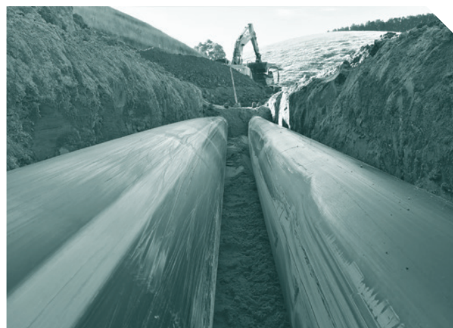
A section of dual pipeline installed near Korumburra as part of the Lance Creek Water Connection.
