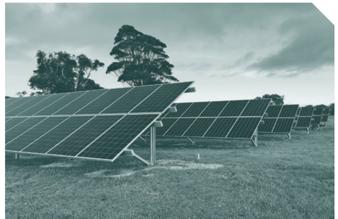
75.6kW Solar system installed at the Lohr Avenue Sewer pump station at Inverloch. It will produce 87% of the sites energy needs.
