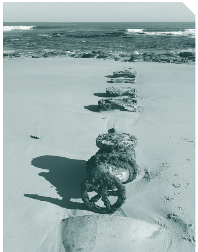
Outfall infrastructure at Venus Bay exposed due to shifting sands.
