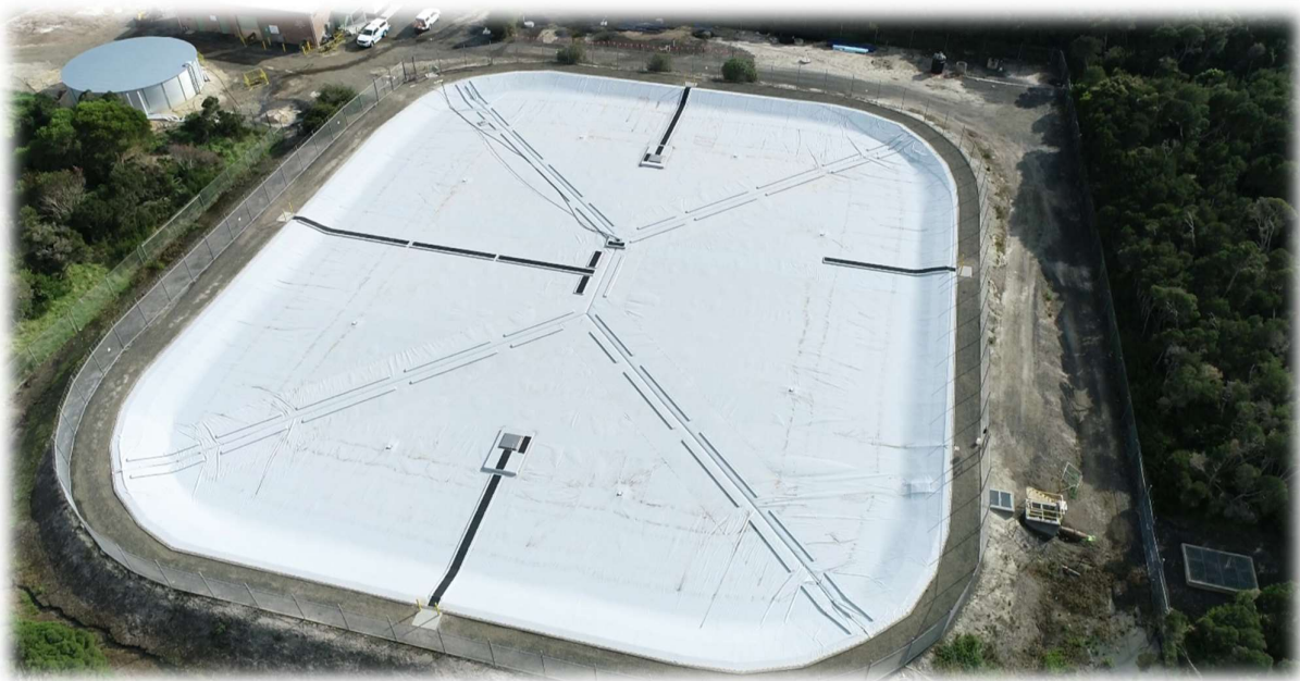
Photo: Wonthaggi clear water storage basin post relining and covering
