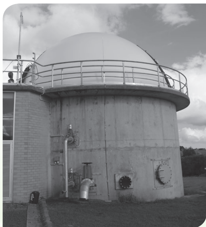
Leongatha Waste Water Treatment Plant anaerobic digester bio dome, constructed during 2013/14.
