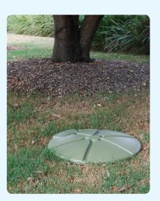
The collection tank lid must never be buried, built over or covered in any way.
