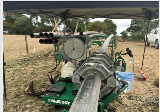
Below: Joining sections of polythene pipe (HDPE)
