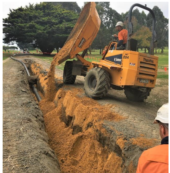
Above: Backfilling pipe trench Korumburra Golf Course. Below: Re-sewing construction corridor to specifications agreed with land owner.
