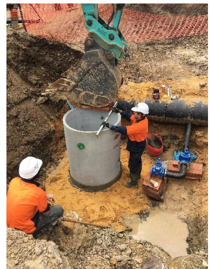
Above: Trench excavation. Below: Installation of a scour valve arrangement.
