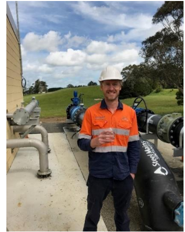
Lance Creek Water Connection’s Chris Hindle takes a moment to sip and reflect on the team’s milestone of water supply to Korumburra.
