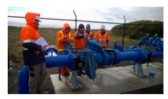
The successful commissioning of the Delivery Point 5 (DP5) valve station and the transfer pipeline connections at the Powlett River and Lance Creek Reservoir have been recently completed. These works will allow for water stored within the pipeline between Cardinia Reservoir and the delivery point to be transferred to the Lance Creek Reservoir.
