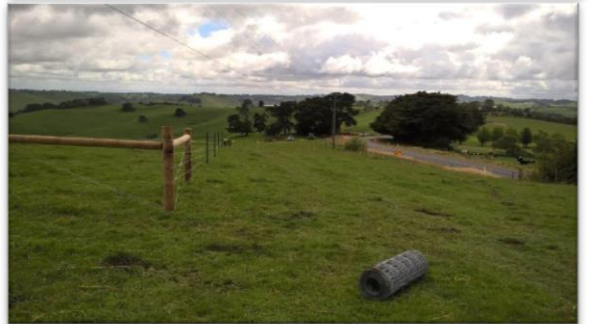
Top – Delivery of high density polyethylene (HDPE) pipe. Middle – Survey work locating existing fibre optic infrastructure. Bottom – Temporary fencing of the construction corridor adjacent to Korumburra-Wonthaggi Road, Jumbunna.
