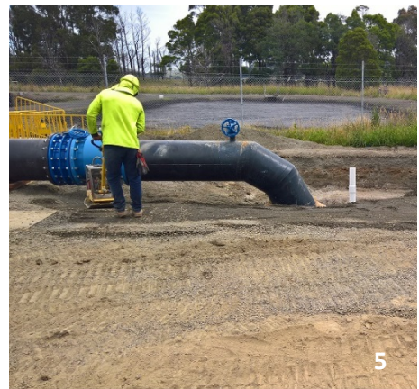
The installation of infrastructure that will connect the new pipeline to the existing storage tank at the Lance Creek Water Treatment Plant.
