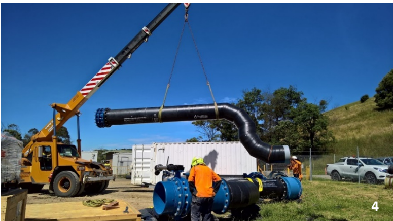
The installation of infrastructure that will connect the new pipeline to the existing storage tank at the Lance Creek Water Treatment Plant.
