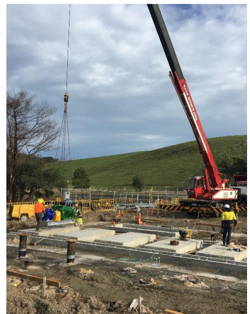
Lance Creek Water Treatment Plant - craning pumps into position before the construction of pump station framework begins.
