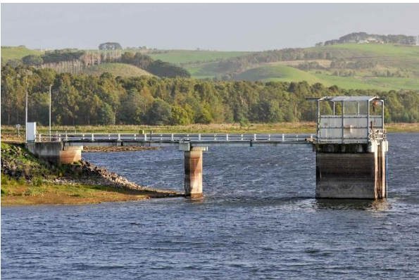
Lance Creek Reservoir water off-take tower
