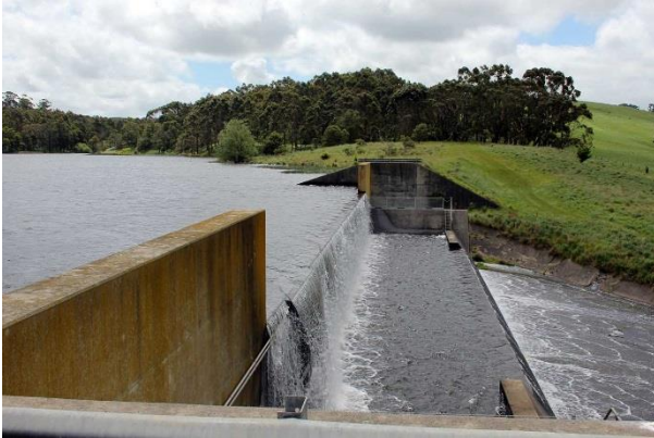
Lance Creek Reservoir spillway
