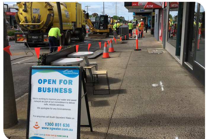
Pictured: Water main upgrade works Bair Street, Leongatha
