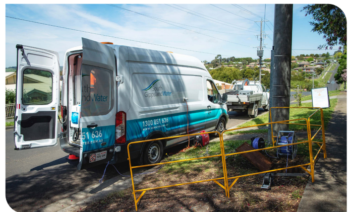
Pictured: The CCTV Van inspecting sewer pipes
